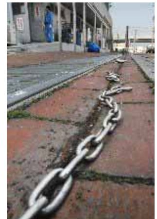
Stainless-steel chain. One part of this was cut and stolen.
